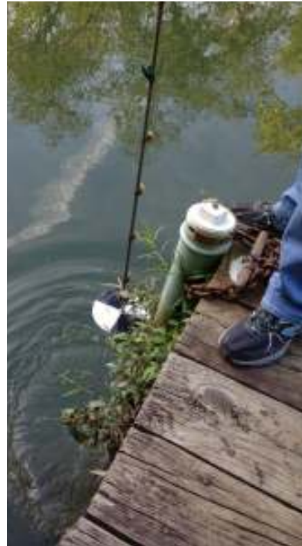
Continuous water quality monitoring station
